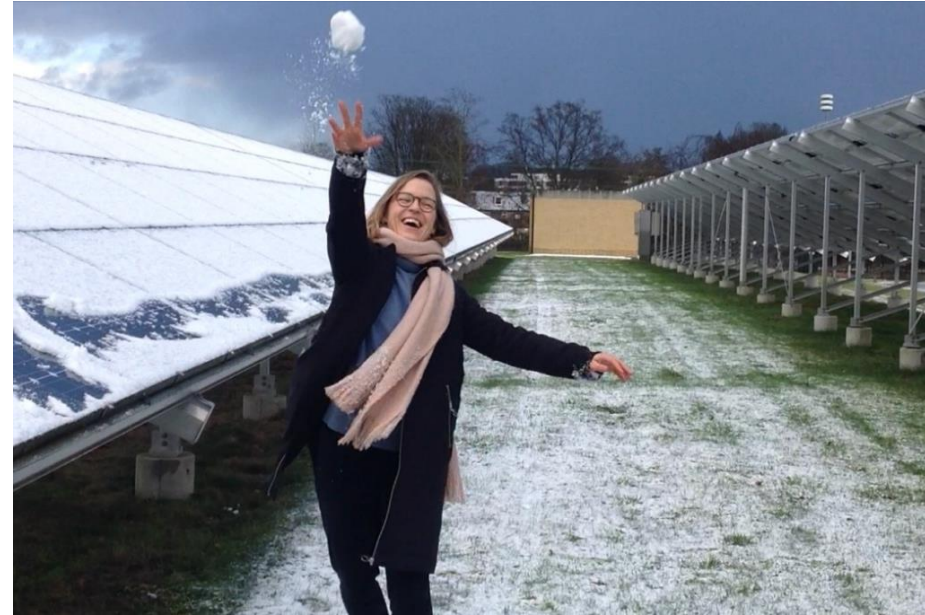
Solar panels at Leiduin in the snow
