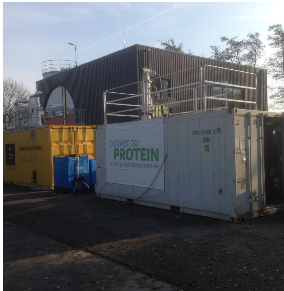
Power to Protein test plant at the Horstermeer wastewater treatment plant
