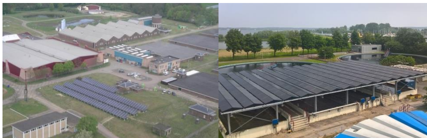
Solar array at Leiduin with 530 solar panels
