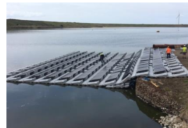
Constructing a floating PV system
