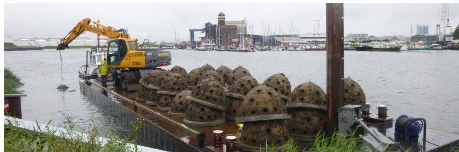
Placing reef baskets in the Noorder IJplas
