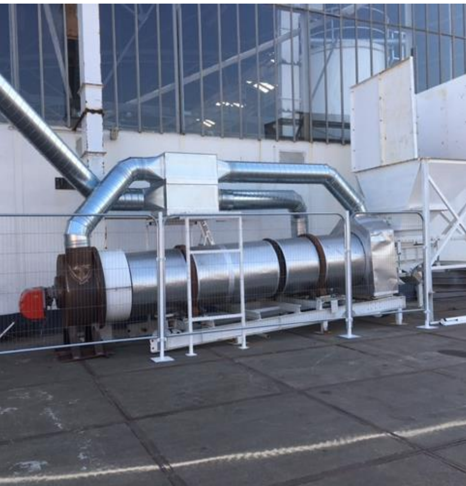
The Calcite Factory under construction
