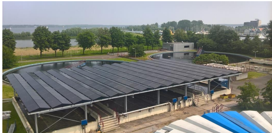
Solar panels on the aeration tank at Huizen sewage treatment plant
