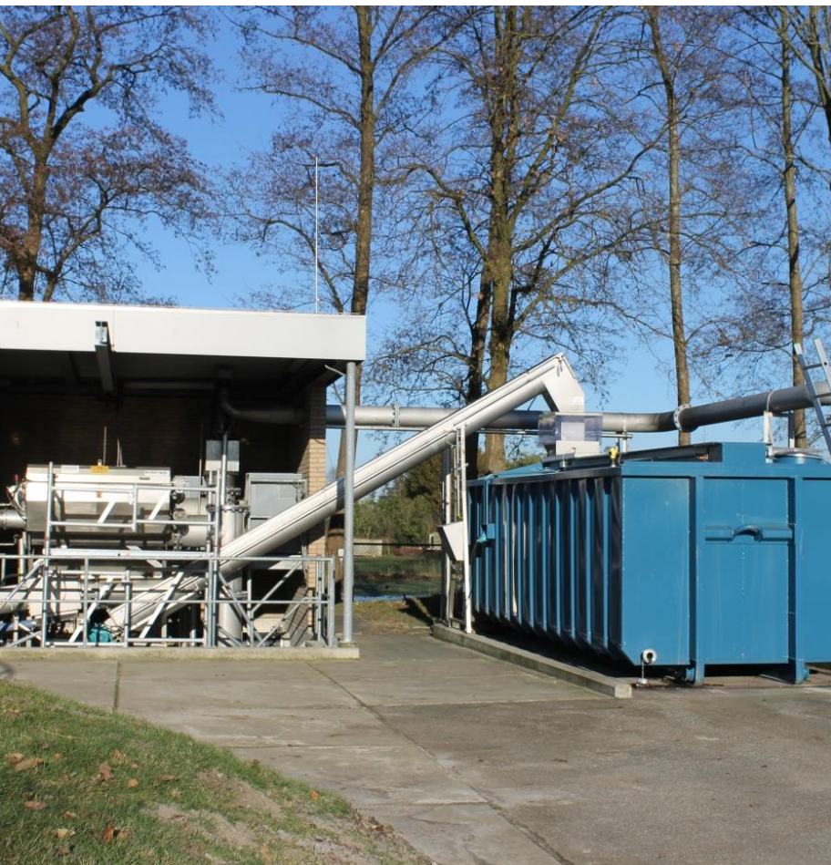
Fine-sieve system at Blaricum STP
